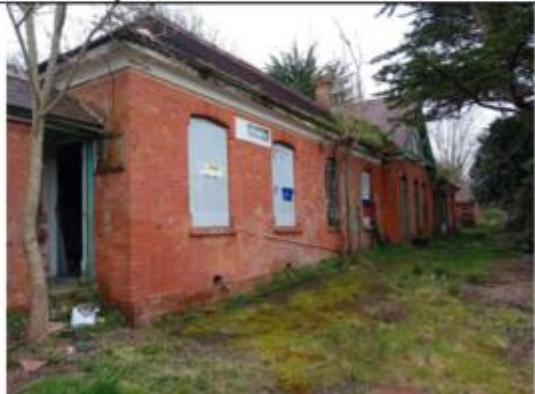
Existing nursery buildings
